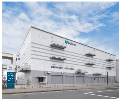
Logicross Yokohama Kohoku
