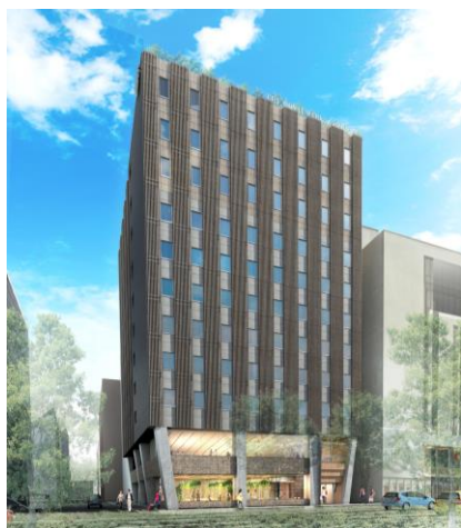
Odori Nishi 1-chome Project
