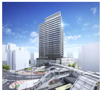
The Parkhouse Hon-Atsugi Tower
