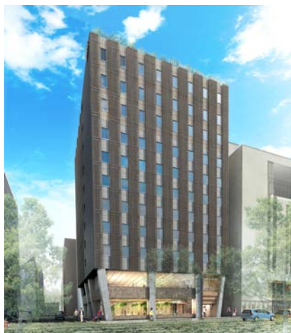
Odori Nishi 1-chome Project
