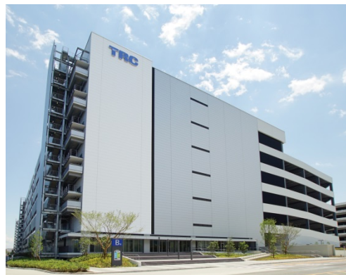
Tokyo Ryutsu Center Distribution B Building
