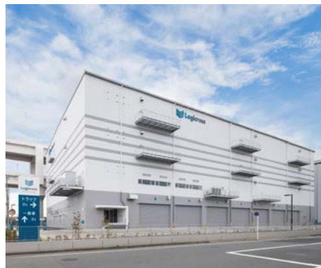
Logicross Yokohama Kohoku
