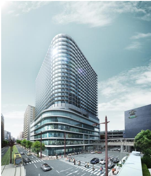
The Parkhouse Kagoshima Chuo Tower
