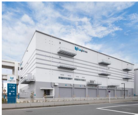
Logicross Yokohama Kohoku
