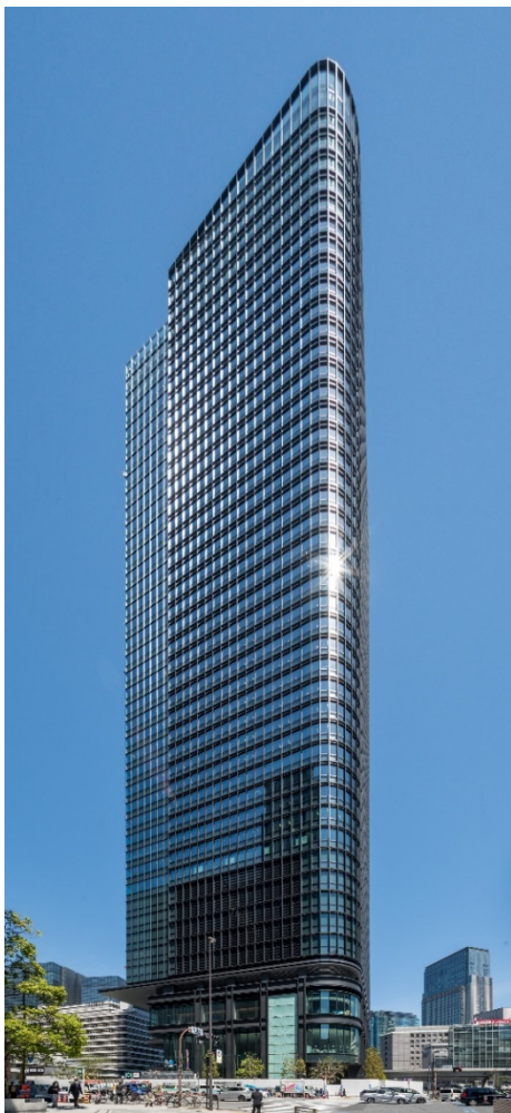
▲ Panoramic view of Tokiwabashi Tower (from the south side of the district)
