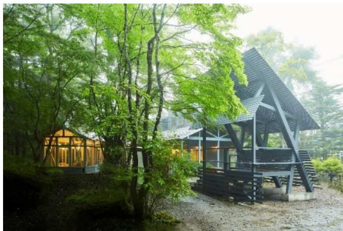
▲「WORK×ation Site 軽井沢」外観
