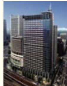
③ Marunouchi Kitaguchi Building (Marunouchi OAZO) Completed in August 2004
