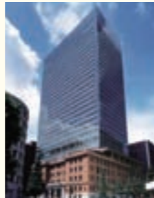
② The Industry Club of Japan and Mitsubishi UFJ Trust and Banking Building Completed in March 2003
