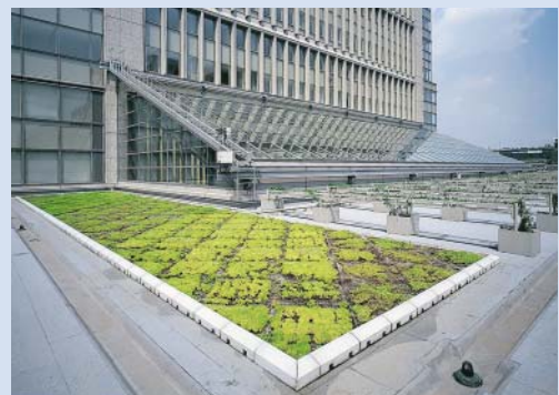
Greenery is planted on the rooftop of the lower level of the Marunouchi Building, helping alleviate the heat island effect.
