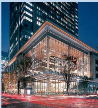
Marunouchi Building atrium “MARUCUBE” (exterior)
