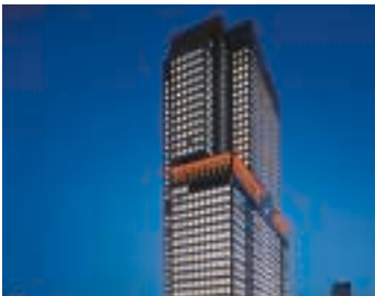
Sanno Park Tower
