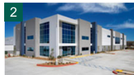
2 Val Verde Logistics Center California Total floor area: 27,000 m 2 Construction completed in 2021
