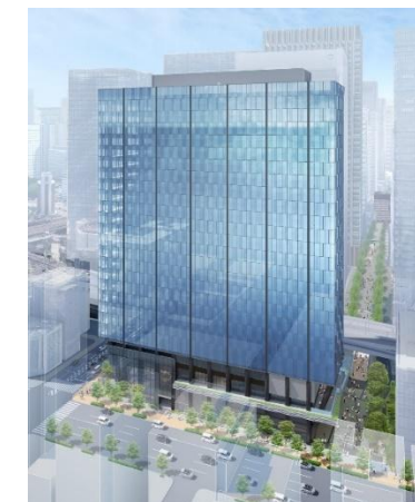
Otemachi Gate Building
