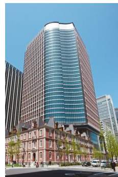
Marunouchi Park Building
