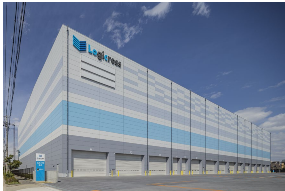
Logikross Osaka Suminoe Completion : Mar. 2025
