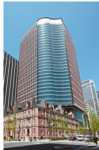
Marunouchi Park Building
