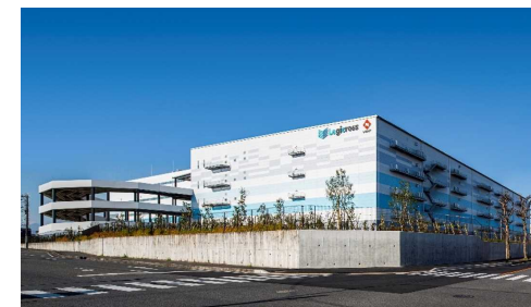
Logicross Sagamihara Completion : Dec. 2023
