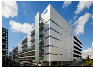
Tokyo Ryutsu Center Distribution A Building Completion : Aug. 2023
