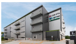
Logista · Logicross Ibaraki Saito (B Building) • Disposed : FY2022
