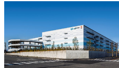
Logicross Sagamihara Completion : Dec. 2023
