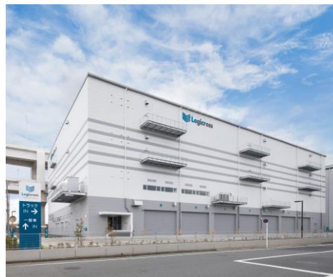
Logicross Yokohama Kohoku
