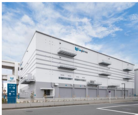
Logicross Yokohama Kohoku
