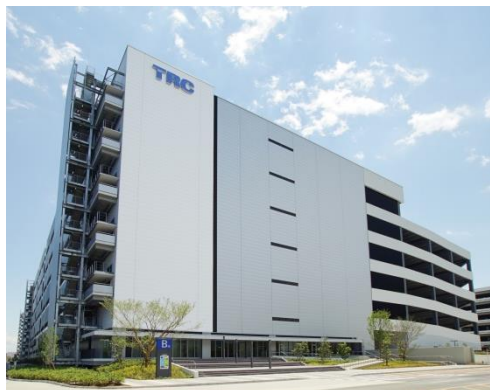
Tokyo Ryutsu Center Distribution B Building
