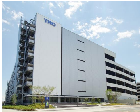
Tokyo Ryutsu Center Distribution B Building
