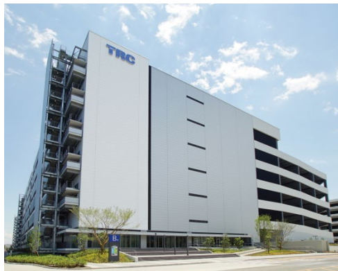
Tokyo Ryutsu Center Distribution B Building
