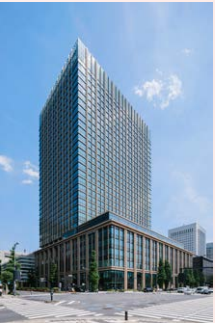
Marunouchi Nijubashi Bldg.
