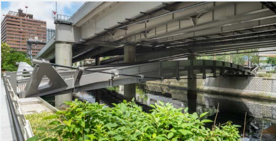
Newly-constructed Nakadori Pedestrian Bridge
