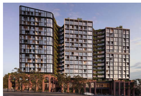
Rozelle Village (Commercial and residential mixed-use development)
