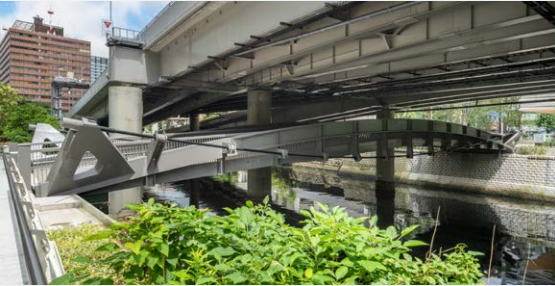
Newly-constructed Nakadori Pedestrian Bridge
