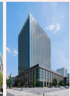
Marunouchi Nijubashi Bldg.
