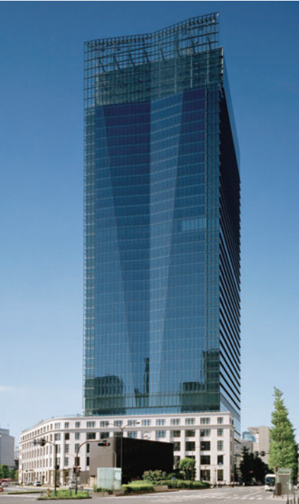
JP Tower JP Tower is a commissioned project for the rebuilding of the Tokyo Central Post Office. Construction on the lower floors involved the adoption of a seismically isolated structure while maintaining a portion of the existing building, while the upper floors have a modern glass façade. As a result, the building creates a new urban landscape that offers a contrast of the old and the new.
