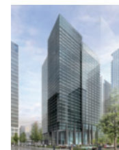
The third phase of the Otemachi Chain Redevelopment Project (Scheduled for completion in fiscal 2017)
